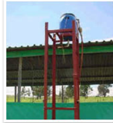
Water Storage Header Tank used for dispensing water + Cell-Vet.
